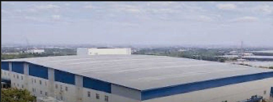
MD HYGIENE MANUFACTURING FACILITY
